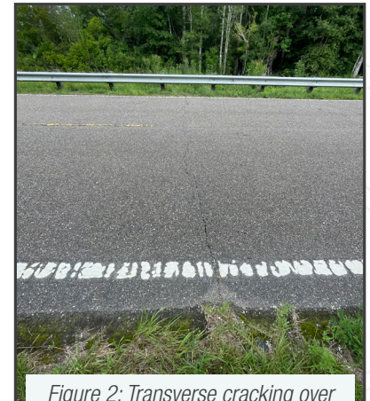
Figure 2: Transverse cracking over existing box culvert
